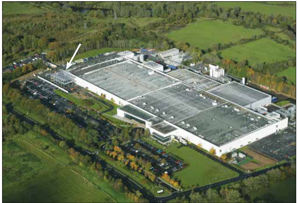
The plant pictured when building work (arrowed) was in progress to increase capacity of TruEye daily lenses
